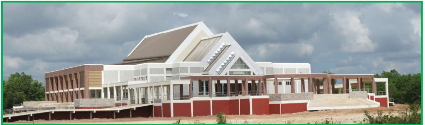
17. AUDITORIUM & SERVICE CENTER BUILDING (TAKSIN UNIVERSITY)
