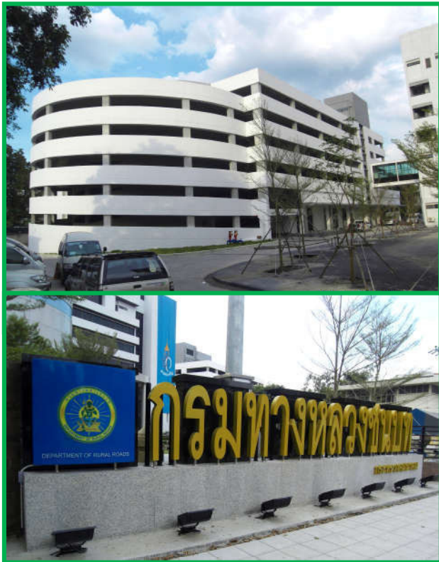
19. HEAD OFFICE CAR PARKING (DEPARTMENT OF RURAL ROADS)
