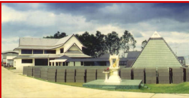
4. CONCRETE ROOF TILE FACTORY (MAHAPHANT CONCRETE ROOF TILE CO.,LTD.)
