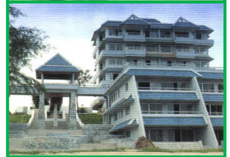
2. EASTERN SEA POINT CONDOMINIUM (CHUENKAMOL RESORT CO.,LTD.)
